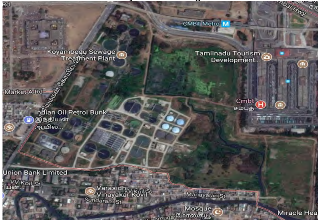
View of Koyambedu Sewage Treatment Plant
