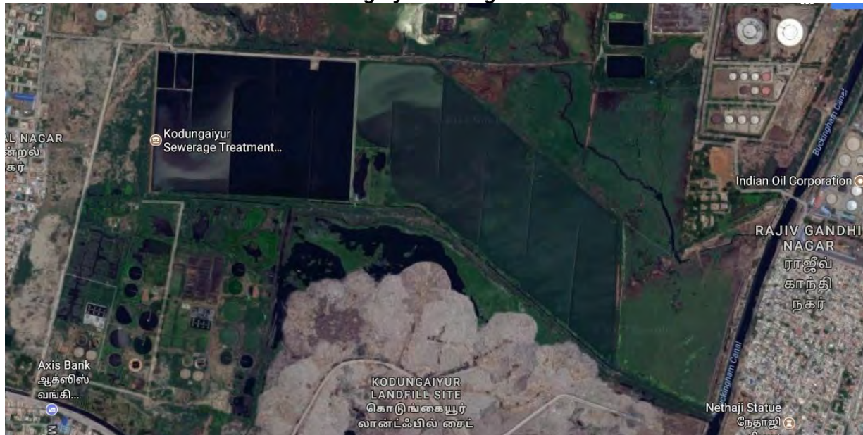
View of Kodungaiyur Sewage Treatment Plant
